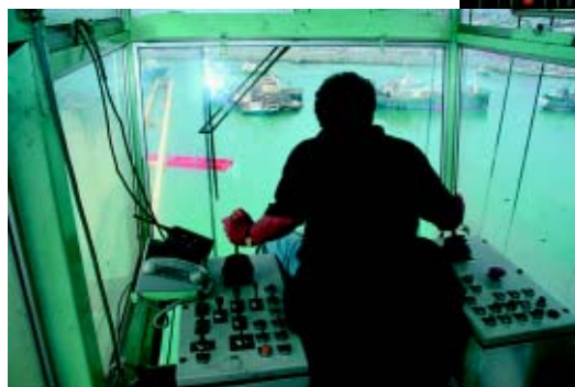
Overhead travelling cranes
