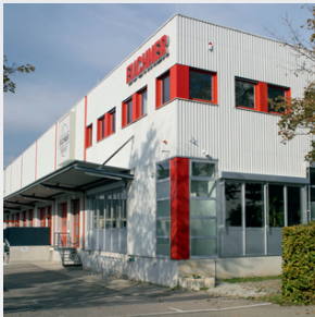
Logistics center in Leinfelden-Echterdingen
